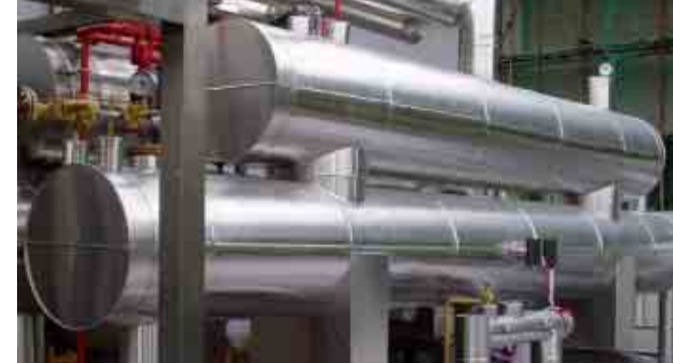
Heat Recovery System-Indirect.
